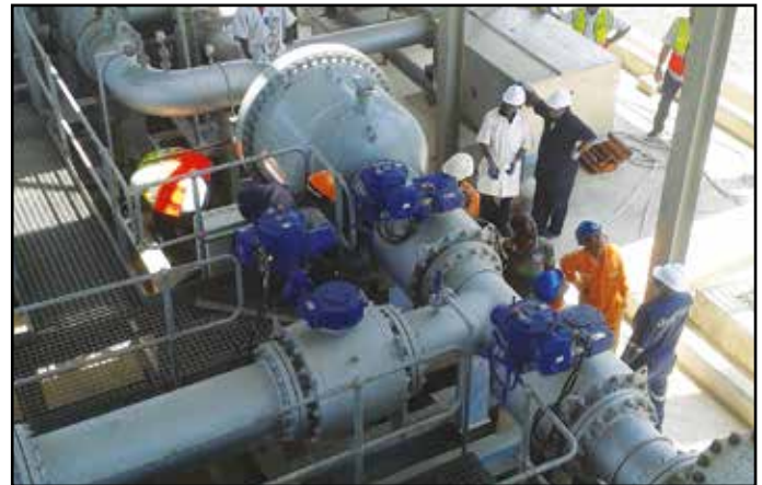
Dual 16" Line Metering Skid
