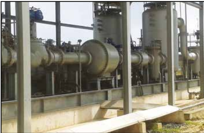
Dual 16" Line Metering Skid
